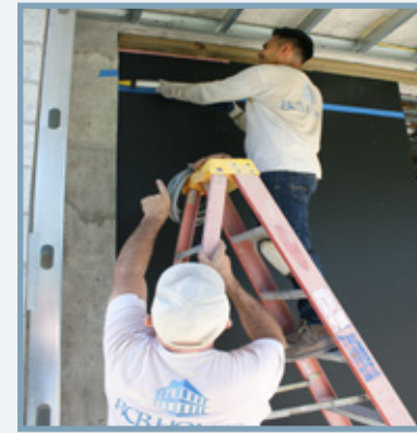
Carlos waterproofing a sliding glass door opening with Leo Murphy
