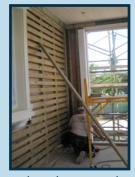
Backing being applied to attach the shingles
